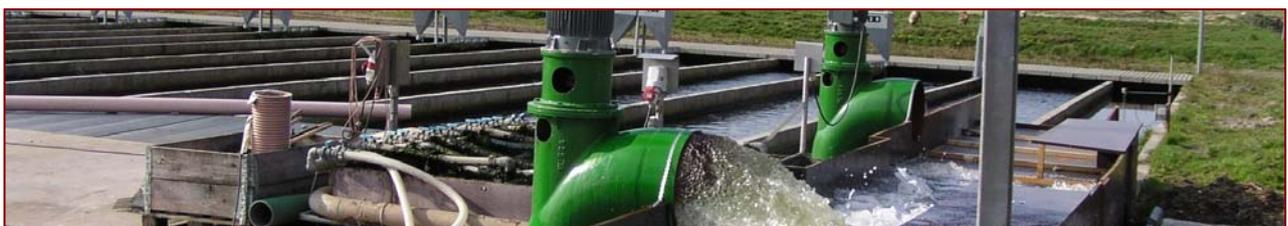
Green LM Propeller Pumps installed in a Danish Aquaculture Plant
